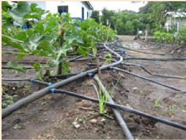
Illustration 6.4: Expensive irrigation system at Diligent's demonstration plot in Arusha.
